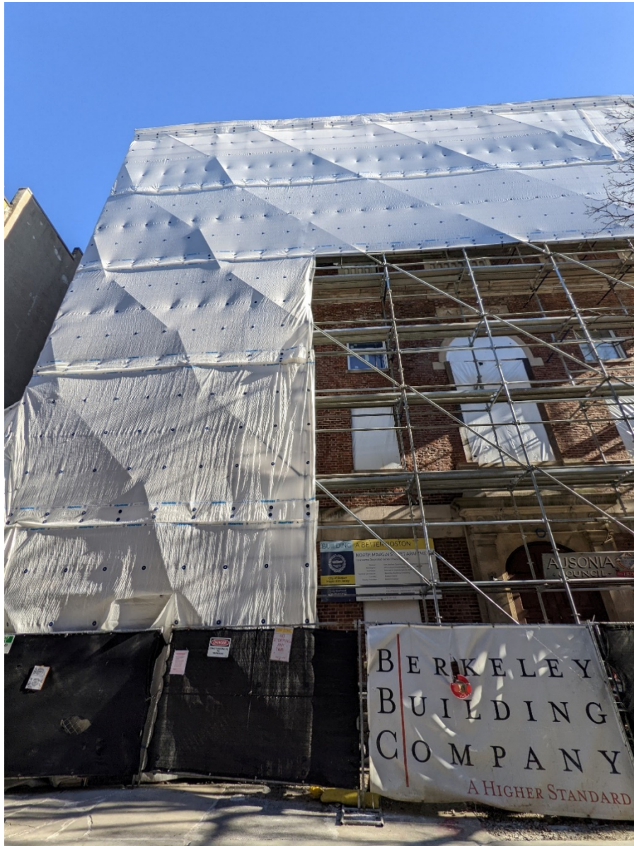
In the North End, CPA funds supported the adaptive reuse of the existing Knights of Columbus headquarters to create 23 affordable apartments for seniors, including three units reserved for seniors experiencing homelessness. This CPA project also developed meeting space for the North End community and acquired a new space for the Knights of Columbus. Source: JM Goldson
