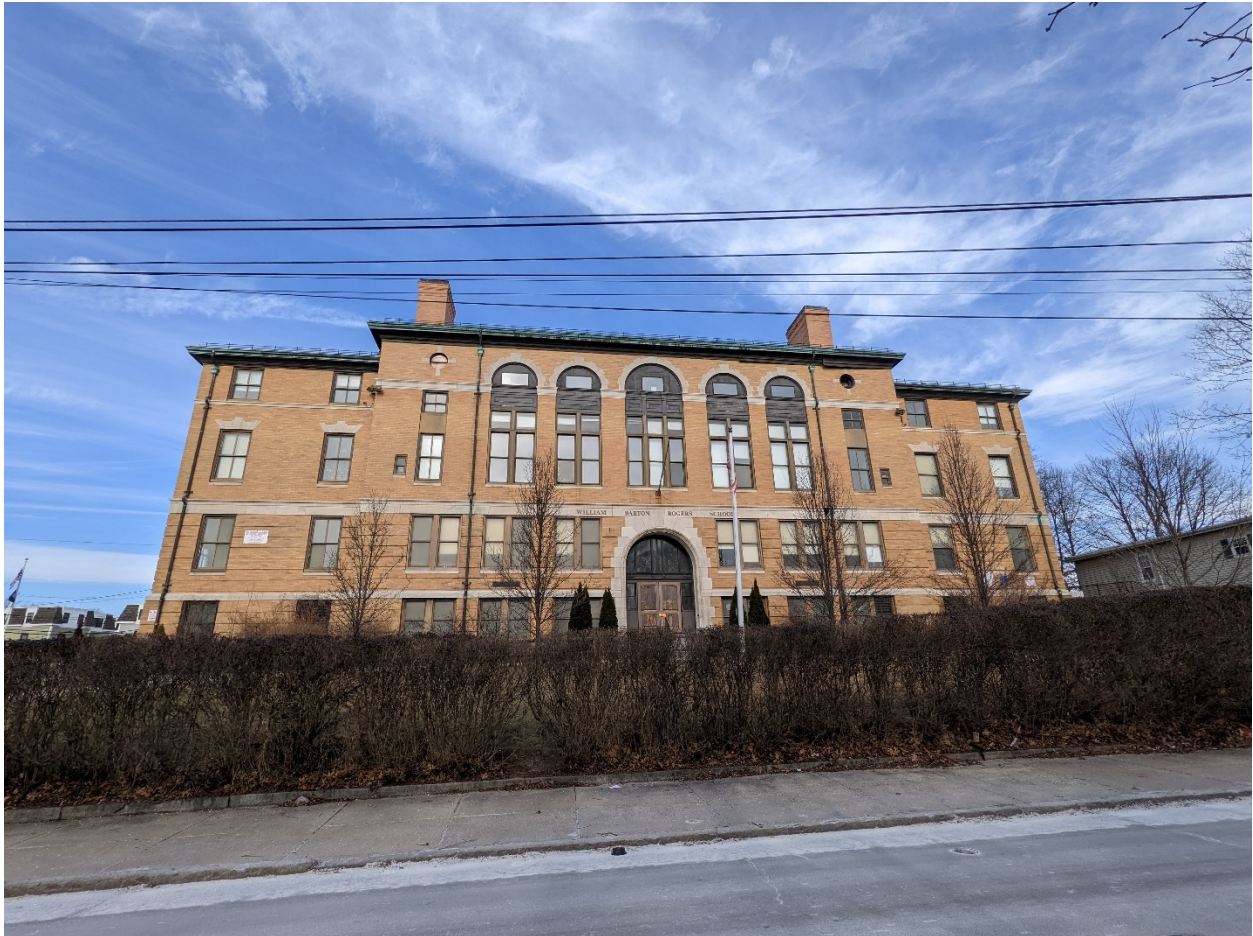
Hyde Park's vacant William Barton Rogers School will be converted into a vibrant, mixed-income, LGBTQ-friendly senior 75-unit housing development through CPA funding. Source: JM Goldson
