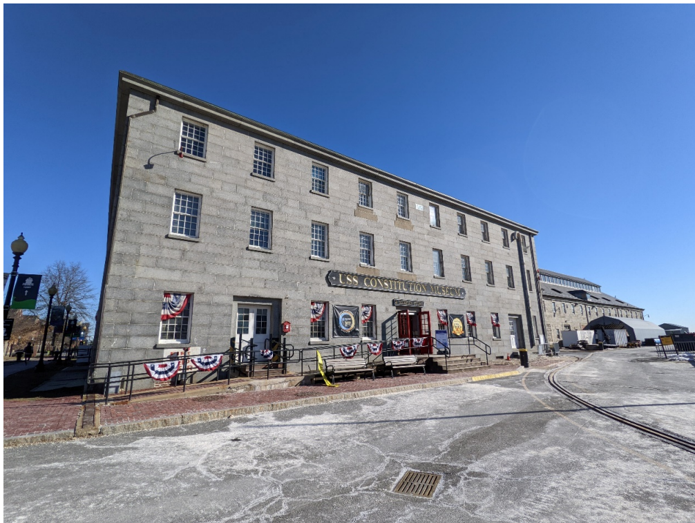
The USS Constitution Museum in Charlestown received CPA funds to relocate the museum's sprinkler system equipment. Source: JM Goldson
