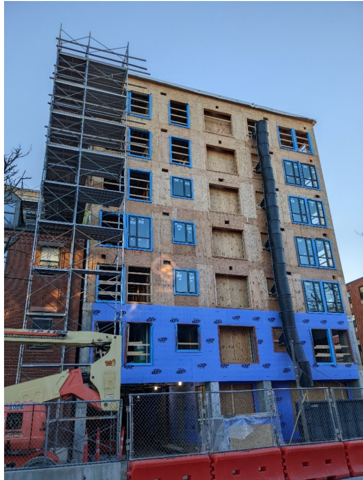
CPA funds are supporting the construction of Grace Apartments in East Boston. When finished, this multi-family development will have 42 units of low-income senior housing, including five units reserved for individuals experiencing homelessness. Source: JM Goldson.
