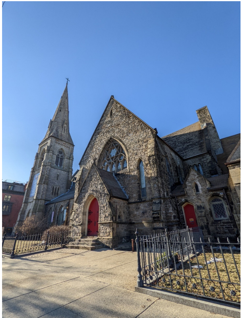
Union United Methodist Church (South End) received CPA funds to finish building a handicap accessibility entrance for the church’s well-used community space. Source: JM Goldson
